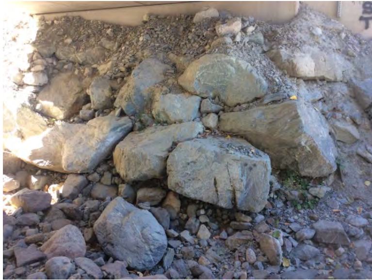
Right Bank Abutment when facing downstream
