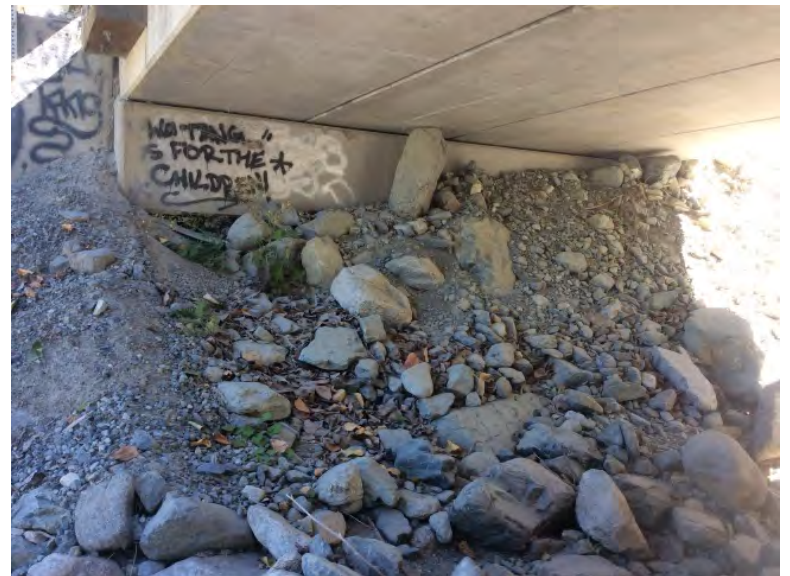
Left Bank Abutment when facing downstream
